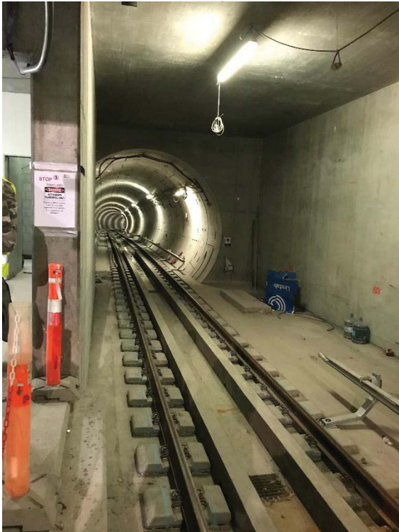
Abbildung 5: U-Bahn Tunnel (Station Nordhavn)
